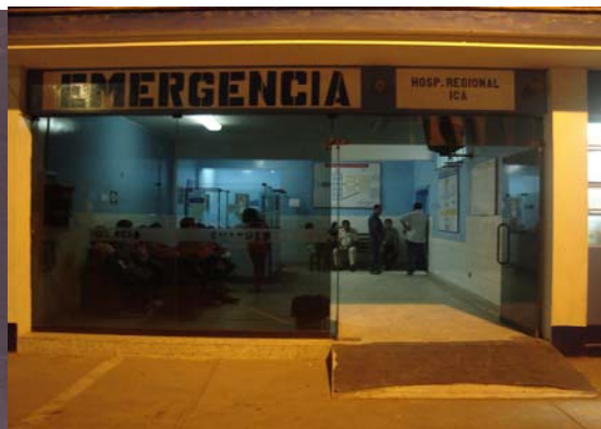
Hospital Regional de Ica.
